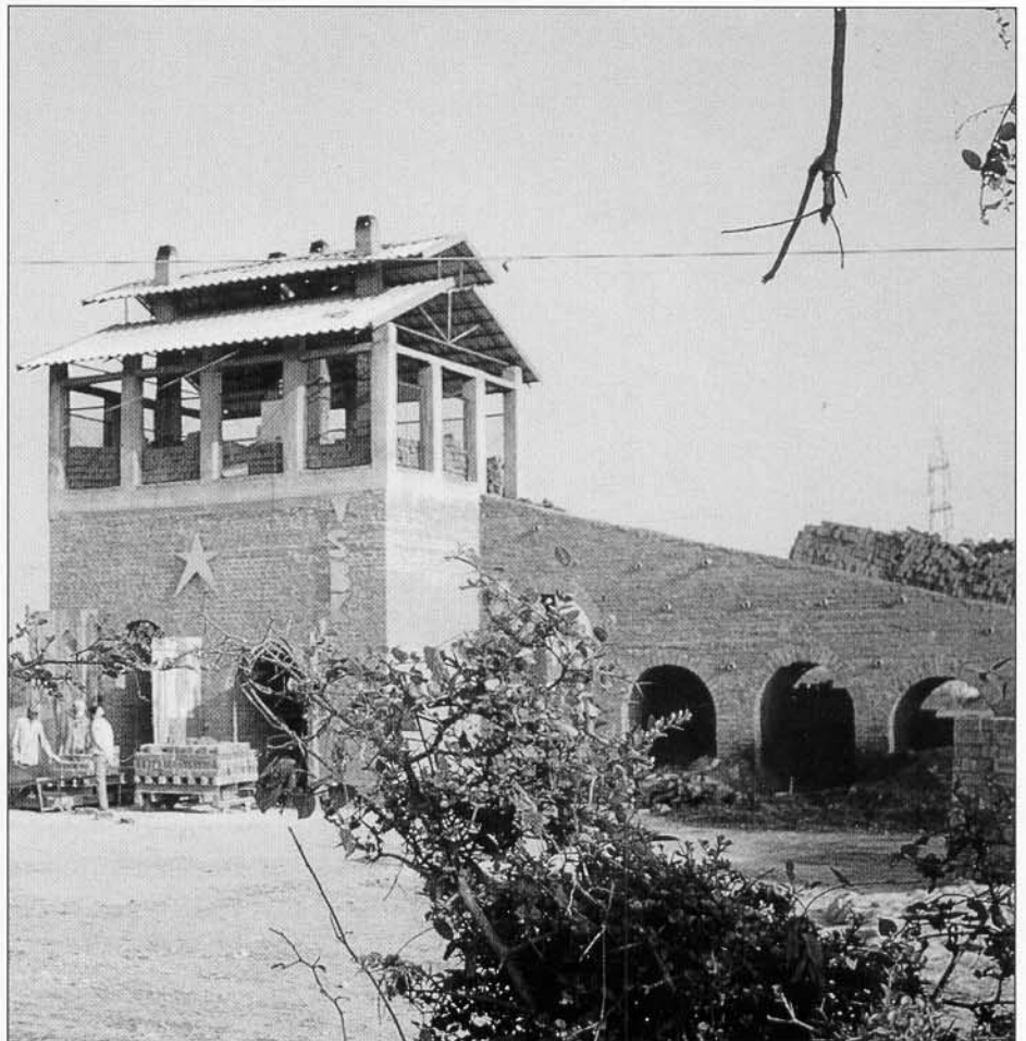
Fig. 8: Kiln after modification
