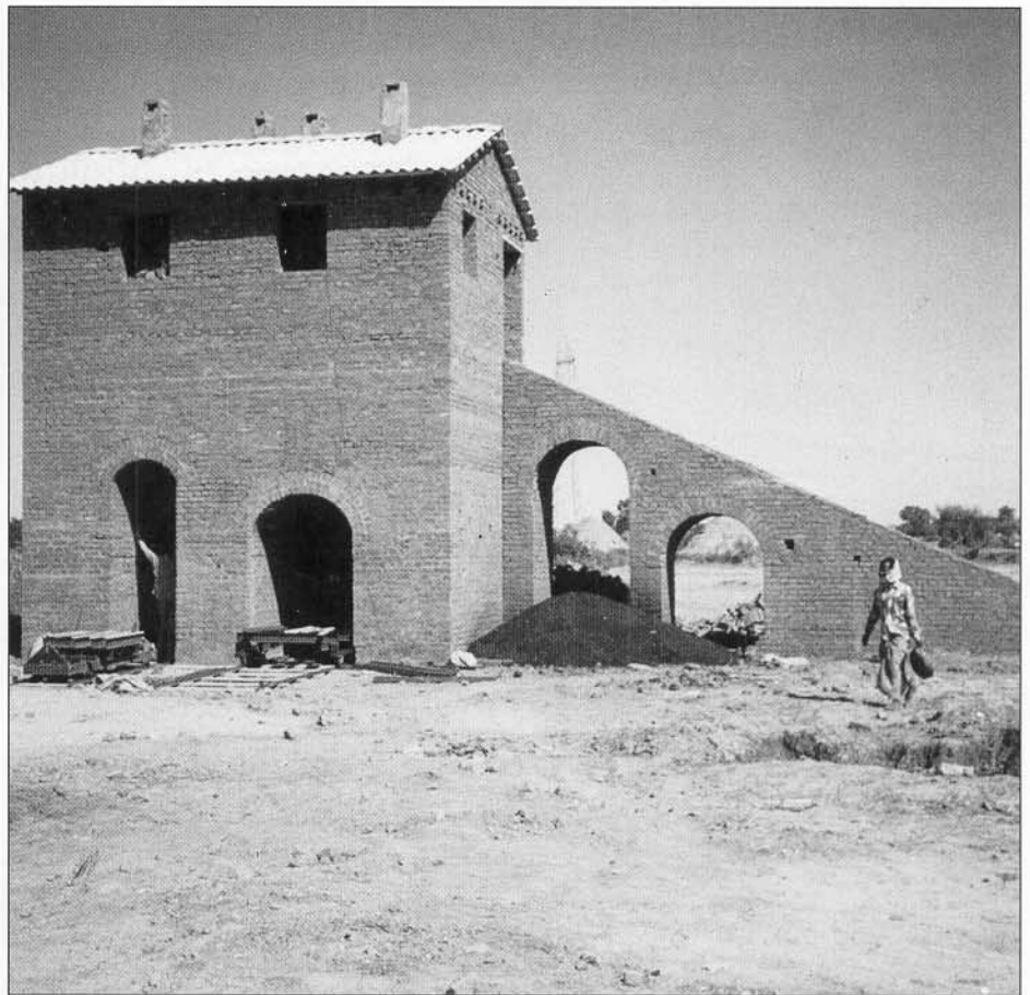
Fig. 7: Kiln after completion of construction before modification
